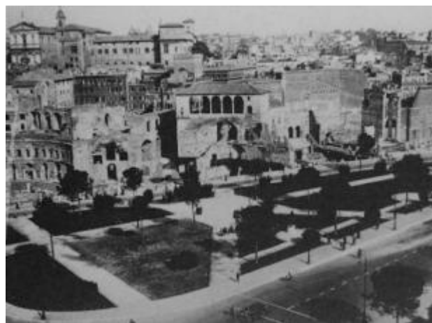
Fig. 7: The area after the demolition. Via dell'Impero was inaugurated on the 1932
