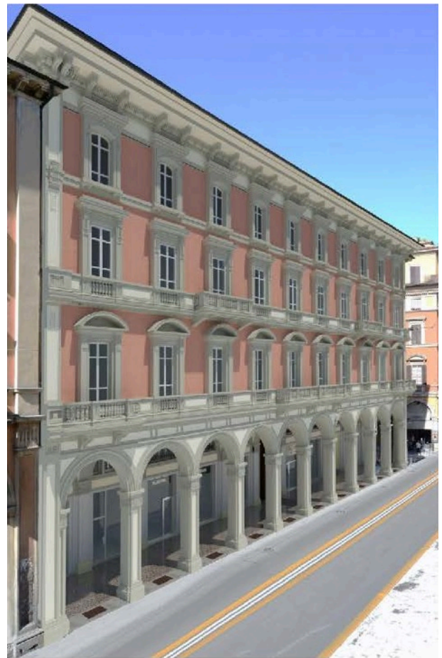
Fig. 9: Huge buildings often have modular elements that repeat themselves along façades. Procedural modeling and geometric instances were explored by students during their training: 3D model by Alice Hecker and Valeria Lenzi.
