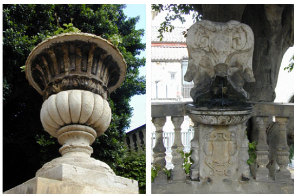
Fig. 7: Stone yard and fountain stone with black crust and biological layers
