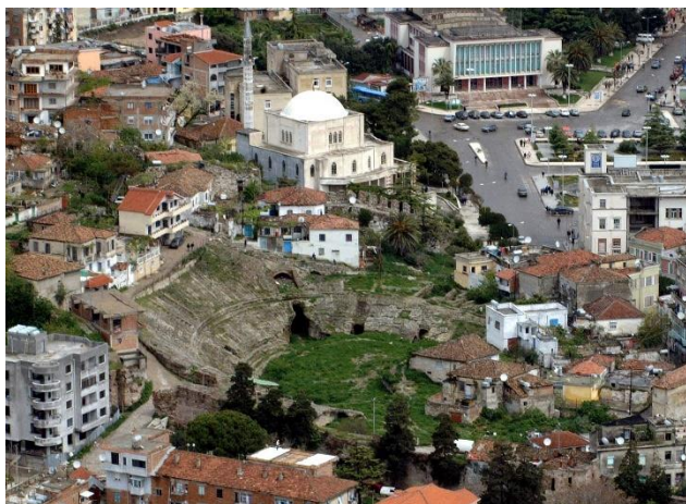
Fig. 1: Aerial view of the amphitheatre and urban fabric from the Ottoman period
