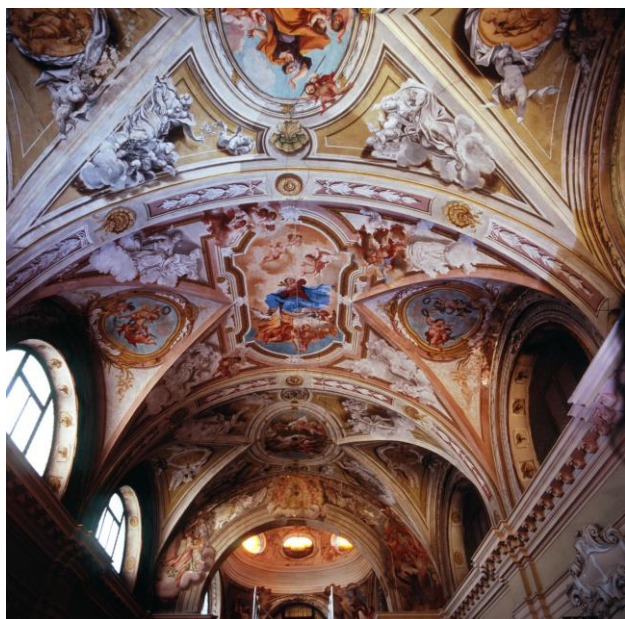
Fig. 1: General view of the frescoed barrel spheroid vault with lunettes of the church of Istituto Sacro Cuore of Trento.
