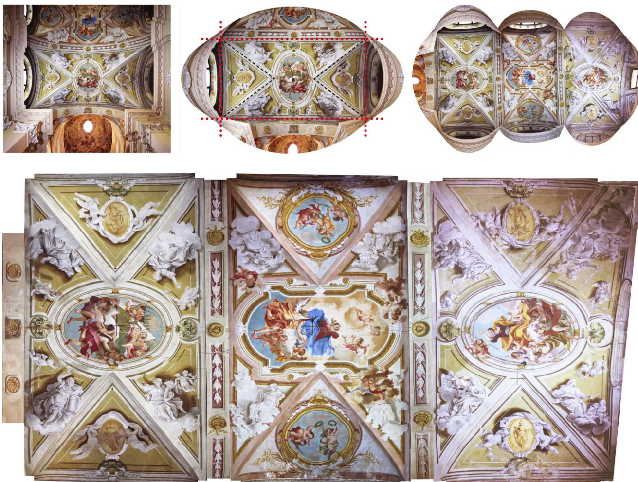
Fig. 4: Transformation sequence of photographs of the vault in a pseudo orthogonal projection.
