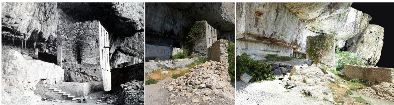
Fig. 5: The west front of the hermitage and the foundations of the church represented in the archive picture, the survey photograph and the orthophoto by 3D scanning.
