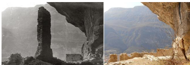
Fig. 4: The ruins of the church in a picture filed in the Historic Photographic Archive in Trento, ca. 1930, and in the corresponding survey photograph, 2014 (Paoli, 2015, p. 103).
