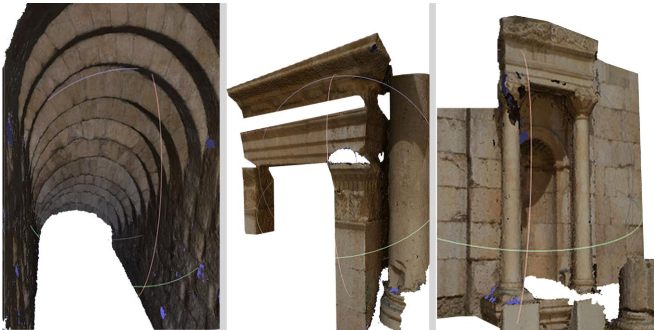
Fig. 6: SfM: construction of details of elements in the theatre in Jerash: a vomitorium, an aedicule of the scaenae frons, a capital
