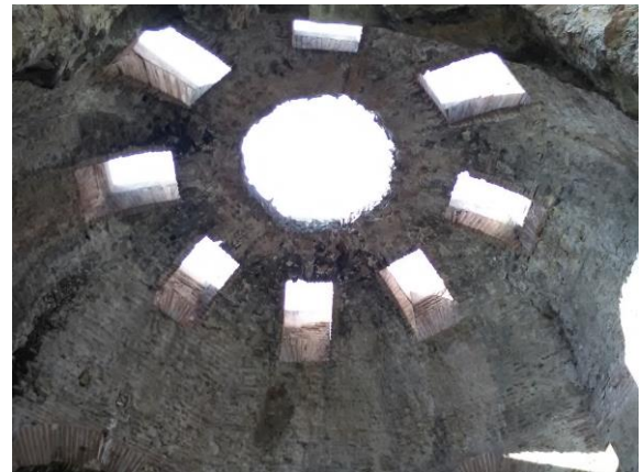
Fig. 7: Nero's Baths in Pisa. Detail of the cloister vault intrados with eight windows and a central oculus on the top. Photo by S. Bertacchi
