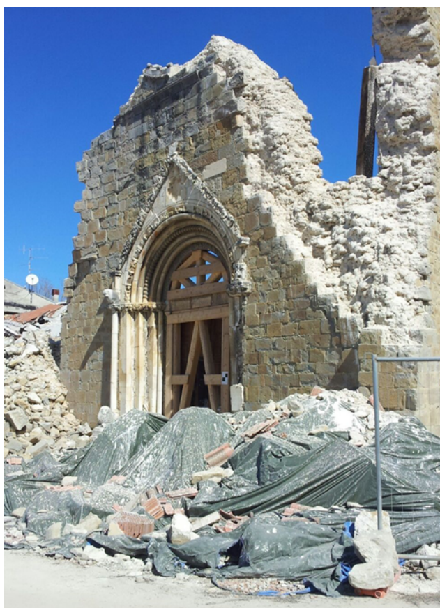
Fig. 2: The ruins of the church of Sant'Agostino of Amatrice, Rieti, after the earthquake of the 24 th August 2016 (photo: C. Mutignani, March 2017).
