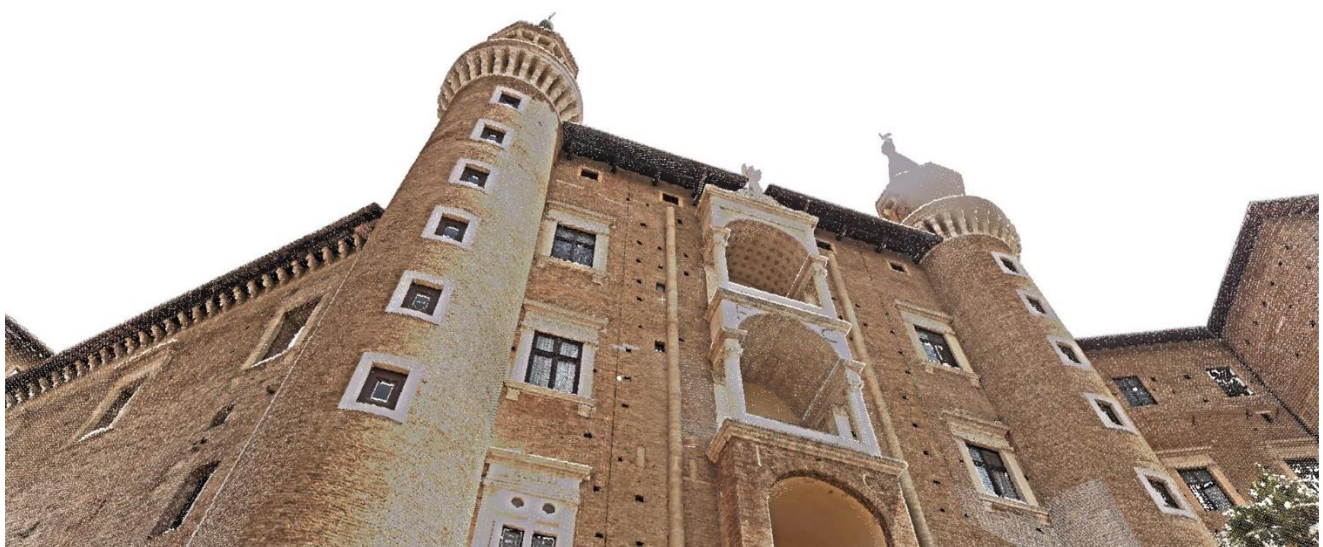
Fig. 1: New point cloud of Laurana's façade with twin turrets.
