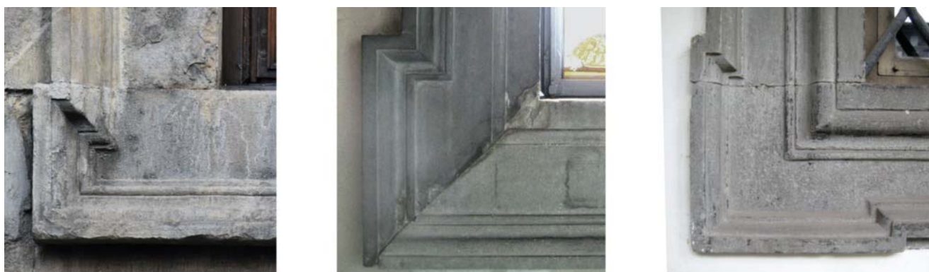
Fig. 1: Comparison of window framing profiles in Florence: Palazzo Bartolini Salimbeni, west facade, ground floor (left); Biblioteca Laurenziana, reading room, inner framing (middle); Santo Spirito, Capella Corsini, Secondo Chiostro (right)
