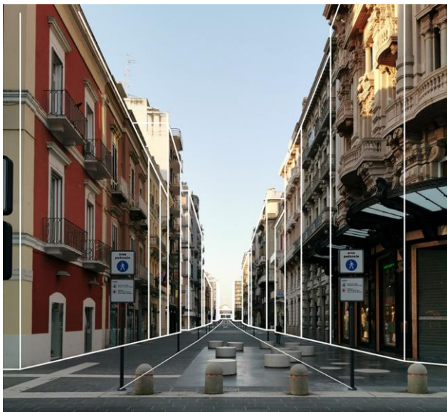
Fig. 5: View of the Sparano street in which the image vertical component is highlighted
