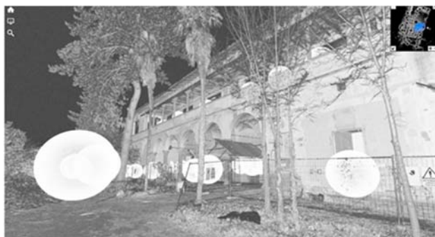
Fig. 16: Scan on the south front
