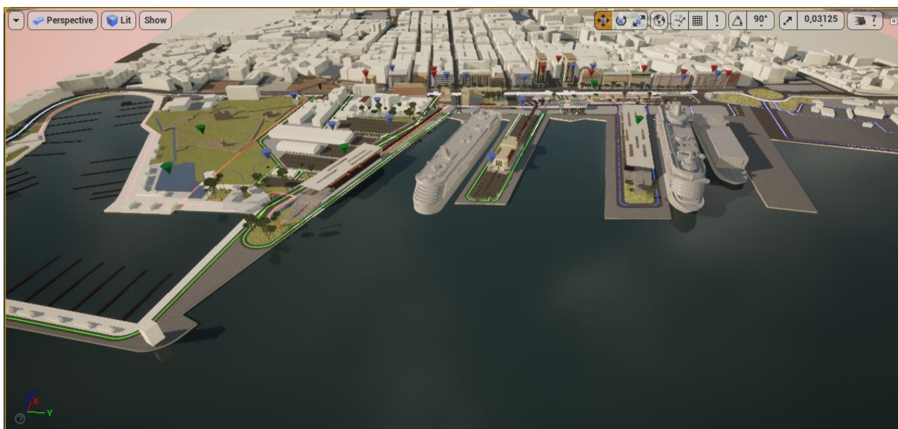
Fig. 13: Aerial view of the virtual model of the project with highlighted flows and services (elaboration by F. Gangemi).
