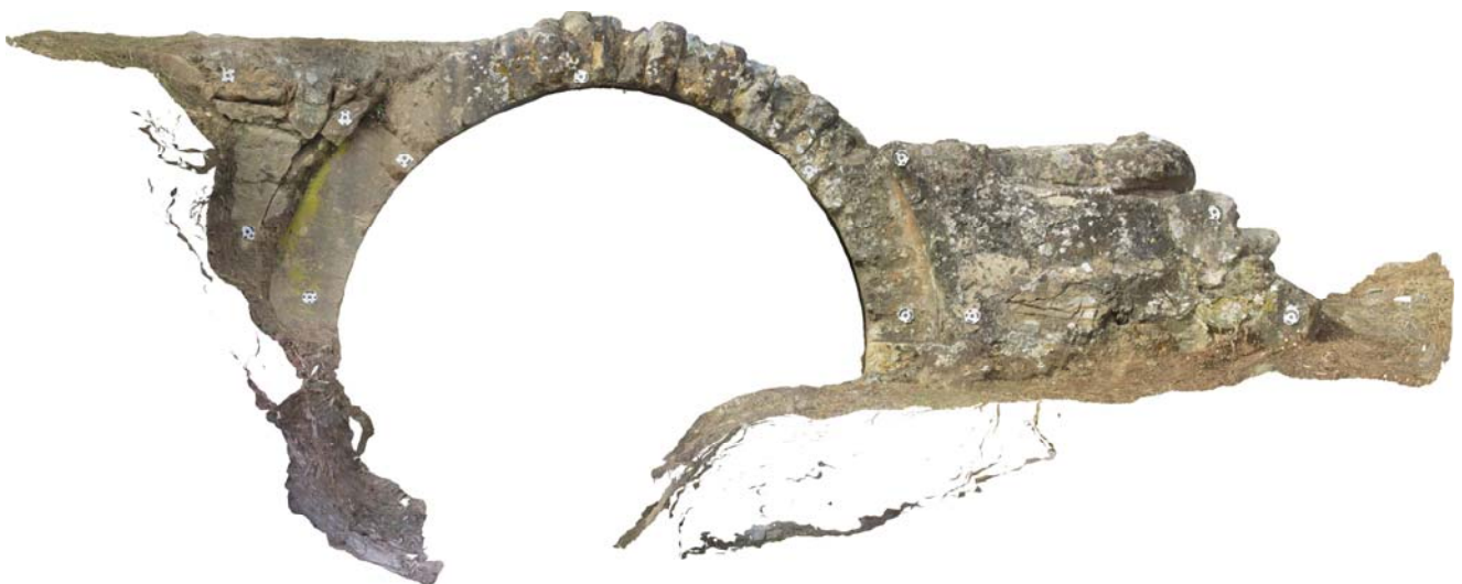
Fig. 4: Photogrammetry of the bridge over the Linares stream (Cordoba). ©Ager Mellariensis/AEI FEDER HAR 77136-R.
