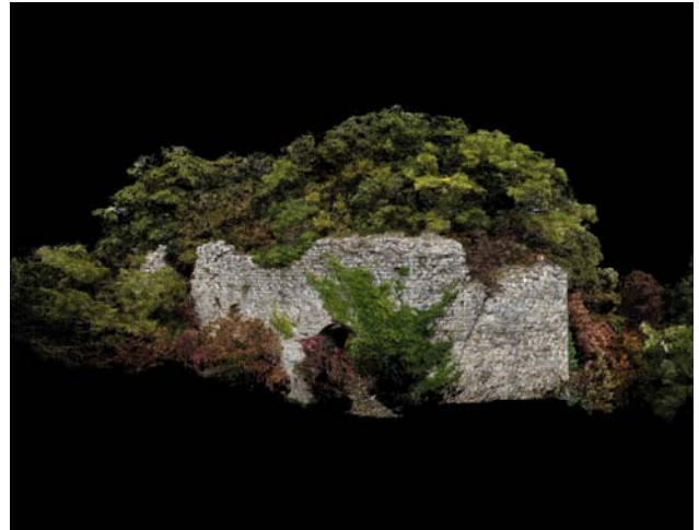
Fig. 3: Remains of the keep and the portal of the castle of San Leolino (photogrammetric elaboration).
