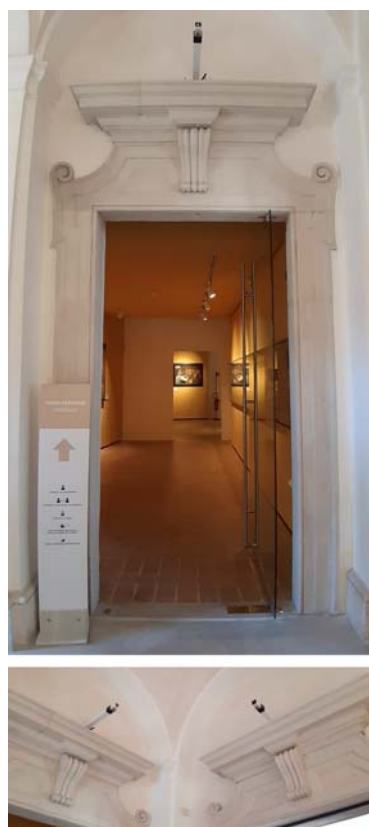
Fig. 5: Re-ID Cameras installed at the entrance and exit of the thematic itinerary on contemporary art.
