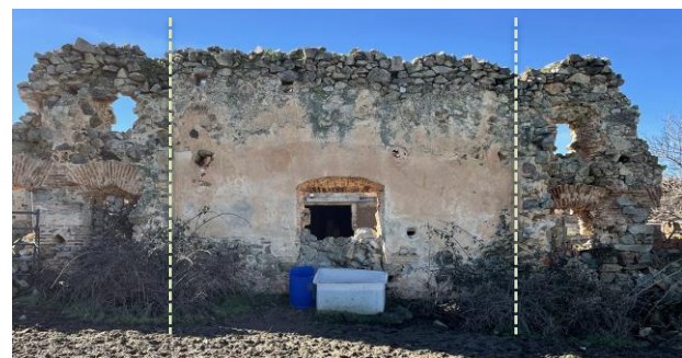
Fig. 5. Difference of historical plastering show old interior spaces. By the author.
