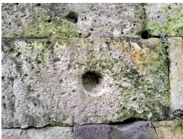
Fig. 2: Picture of one of the marks still visible on the stone ashlars of the city walls caused by a stone ball hurled by the besieging army. Credits: S. Gonizzi Barsanti
