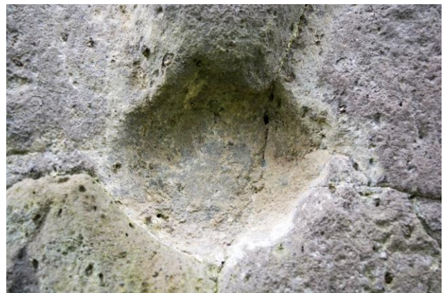
Fig. 5: One of the marks still visible on the tufa ashlar of the city walls caused by a stone ball hurled by the besieging army. Credits: S. Gonizzi Barsanti
