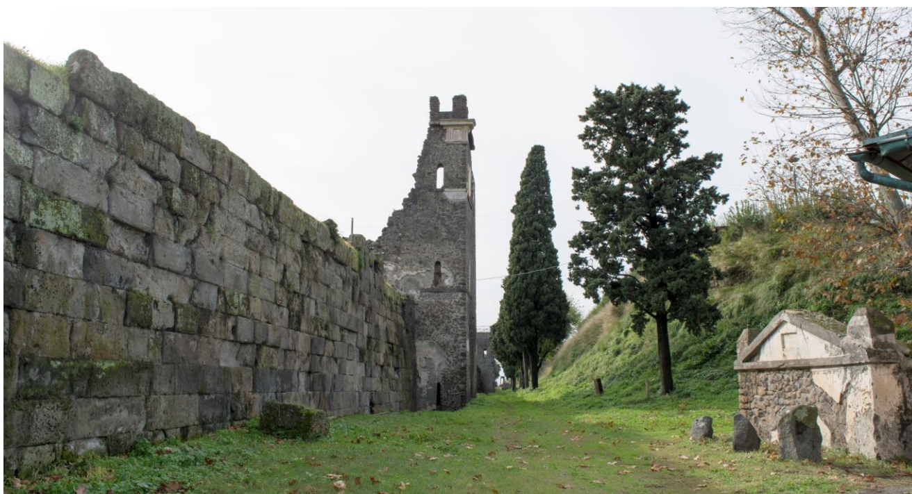
Fig. 1: The northern city walls of Pompeii, seen from the Vesuvio Gate towards Tower X. Credits: A. Rossi
