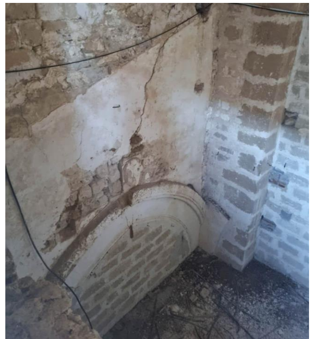
Fig. 8: View of the eastern wall of the presumed dismissed transept: remnants of the pointed arch of the lateral chapel.
