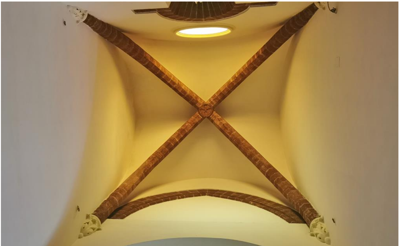
Fig. 9: View of the eastern cross-vault of the lateral apse and pointed arch.
