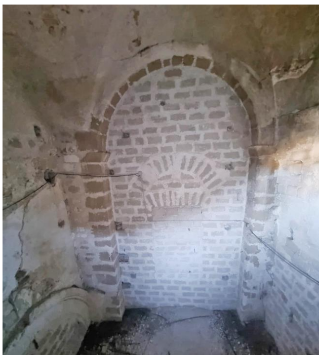
Fig. 10: View of the wall separating the presumed dismissed transept from the tribune: walled-up arch and traces of the blind window.
