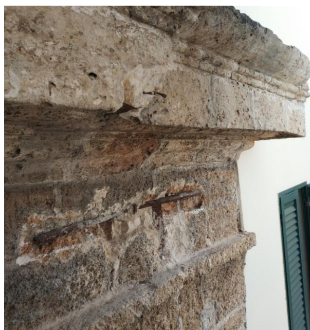
Fig. 28: East elevation, oxidized key head of a chain
