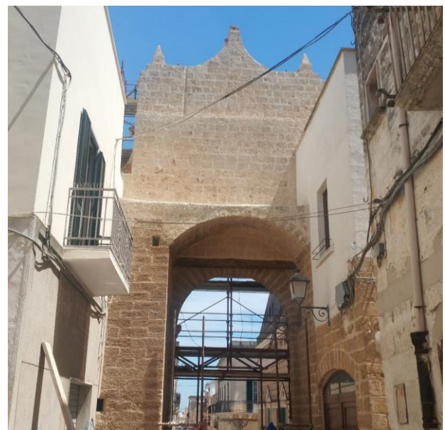
Fig. 37: Ovest elevation, after completion of the works
