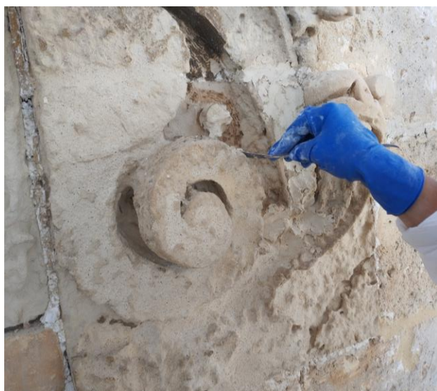
Fig. 32: Grouting of alveolized surfaces
