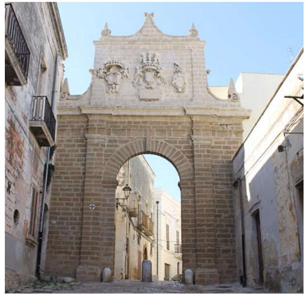
Fig. 35: East elevation, after completion of the works
