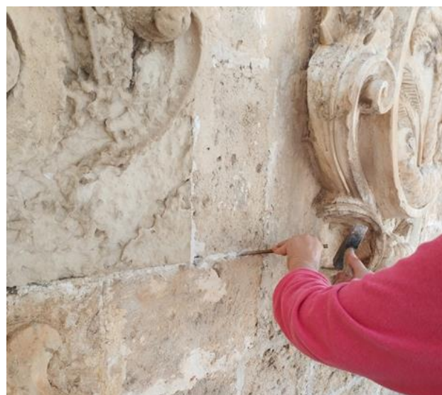
Fig. 33: Removal of improper grouting with chisel
