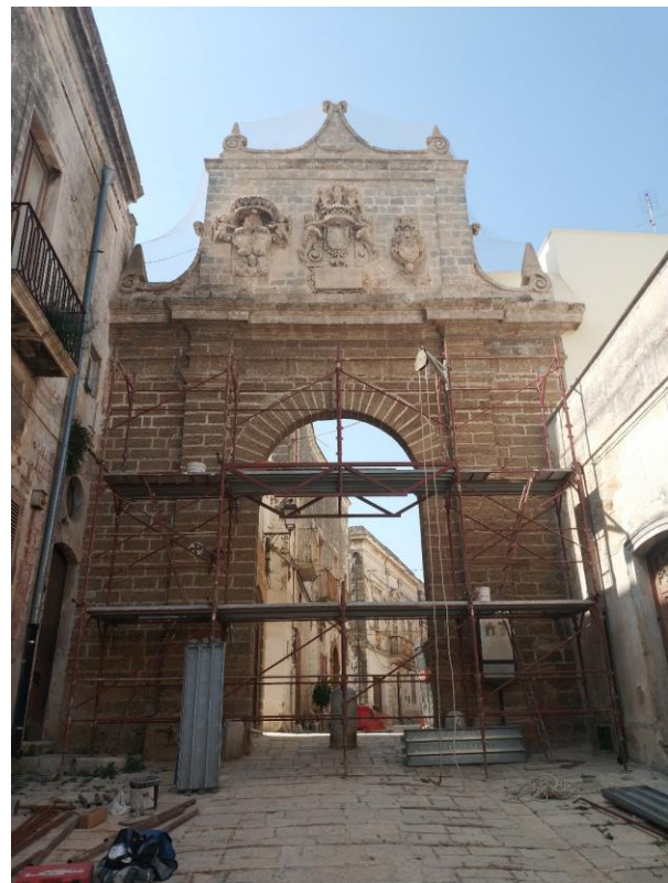
Fig. 20: East elevation, state of the site before the intervention
