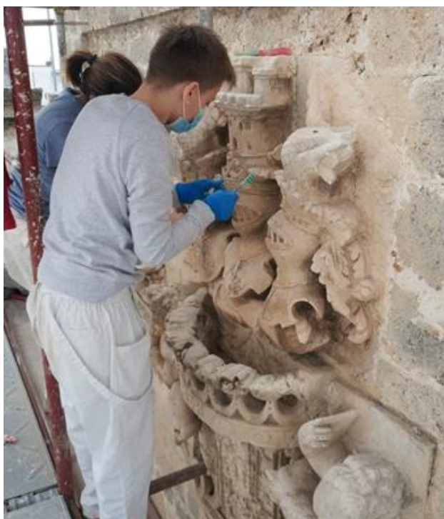
Fig. 30: Cleaning operations of the sculptural modelling
