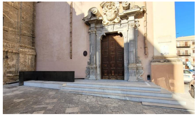
Fig. 8: The new churchyard with the ramp, planned and realised in 2021 in the church of S. Maria in Valverde in Palermo thanks to the 'I-Access' project (photo by C. La Mantia, 2022).
