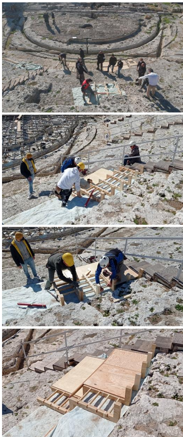
Fig. 7: Test and in-situ assembly phases of the prototype
