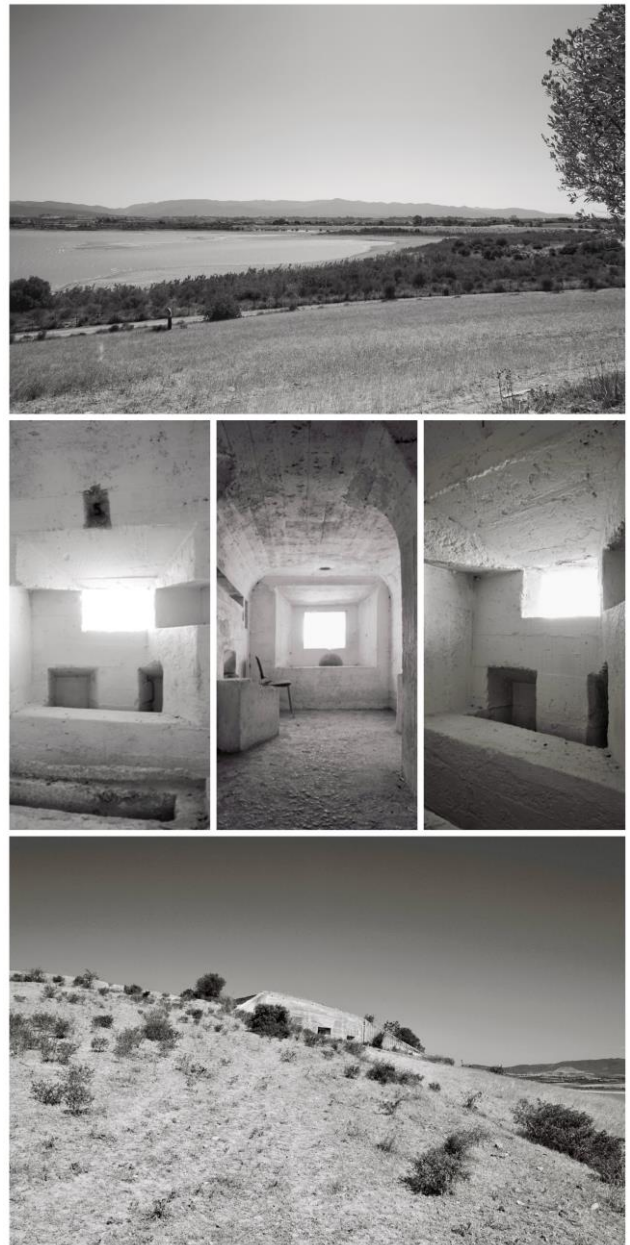
Fig. 25: Collage of photographs documenting Bunker No. 25, part of the Licata stronghold. From top to bottom, the images show: a panoramic view of the Simbirizzi Lake landscape from the roof of position No. 25; the three embrasures, respectively for a heavy machine gun, an anti-tank gun, and a heavy machine gun; and finally, an external view of the fortified position highlighting its location on the hill adjacent to the lagoon (photos by the authors 2024)
