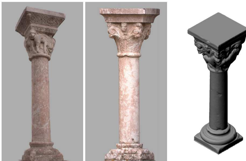
Fig. 3: Results of the points cloud and the polygonal mesh of columns using multi-stereo correlation protocols.
