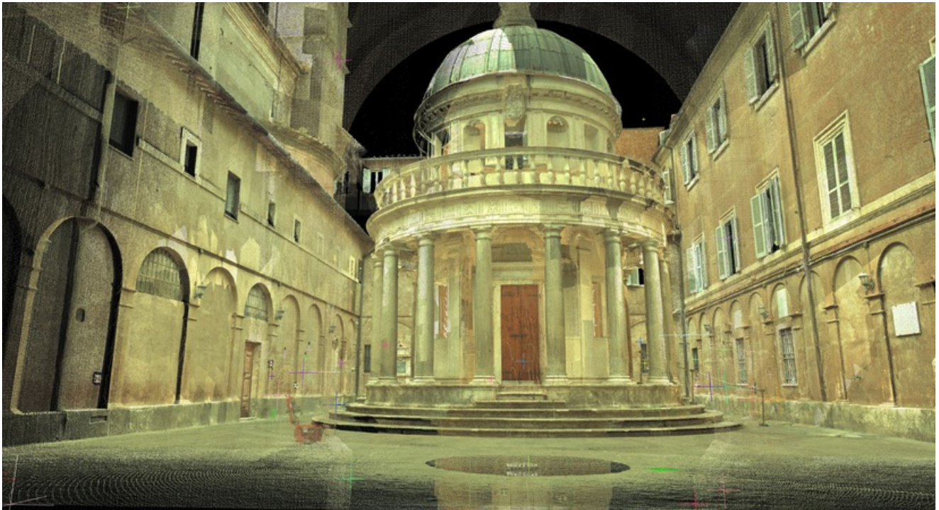
Fig. 2: The Tempietto of San Pietro in Montorio (Rome): data acquired using 3D scanning.
